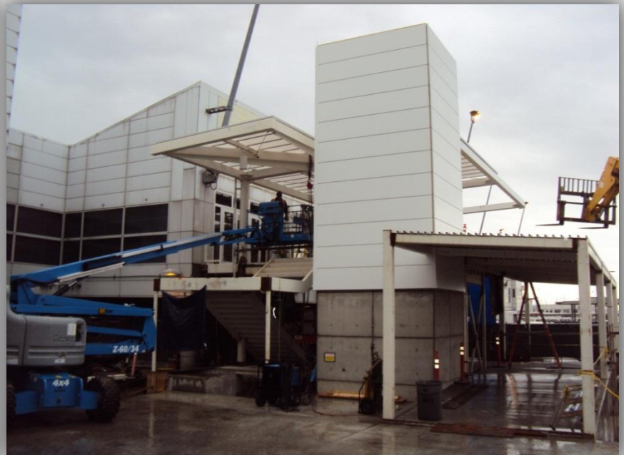
C10 Phase 1 Lobby, Elevator Shaft & Walkway
