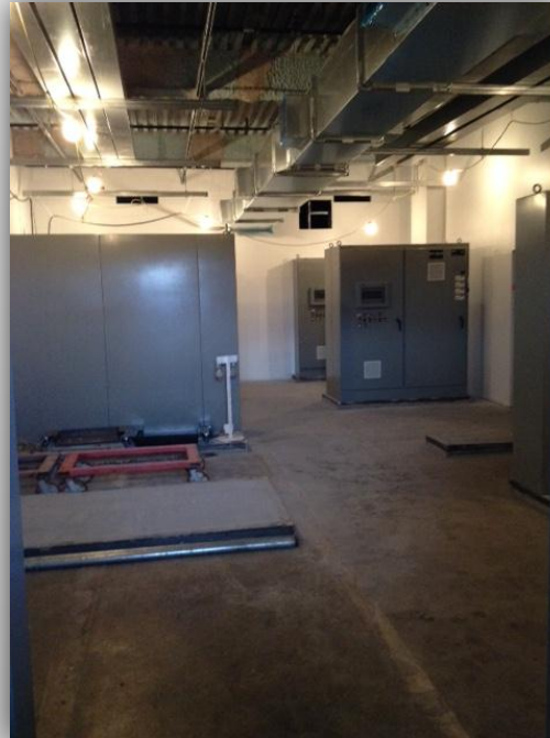
C88 Motor Control Panel Room Construction Progress
