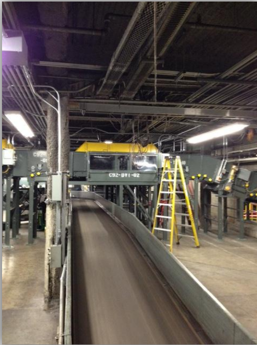
C92 Mainline 1 Conveyor back in operation
